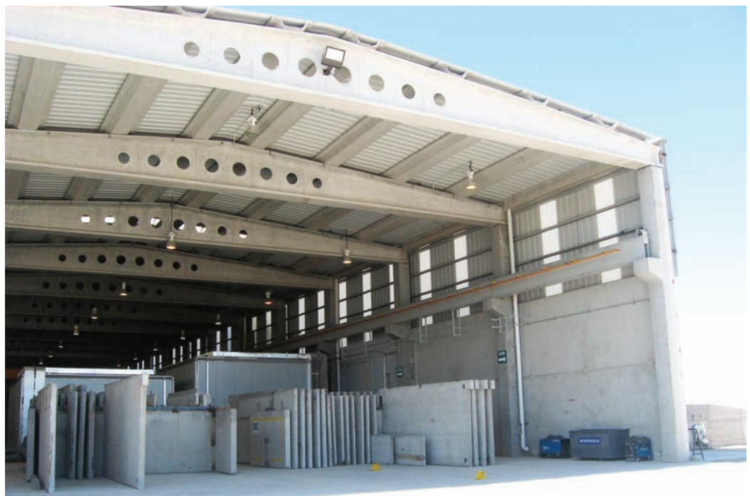
Finished product storage after second stage curing
