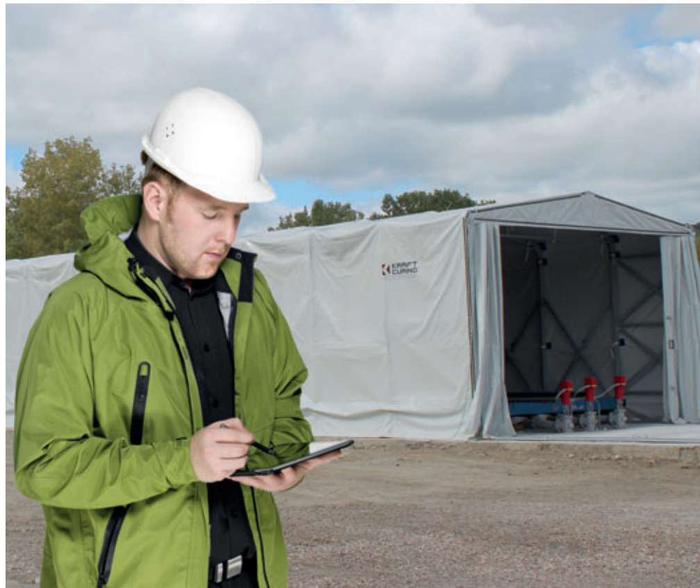
The VaporWare system allows for control and manipulation of all curing procedures over the internet.
