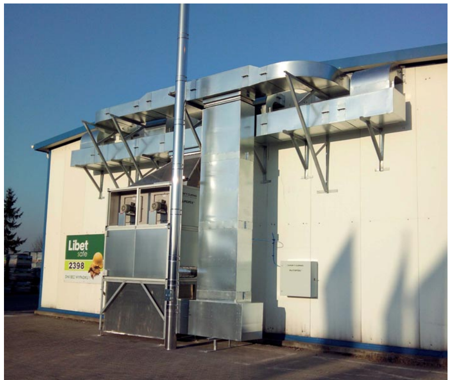
The complete Quadrix® system was installed at the rear of the insulated curing chamber. This system was equipped with an enclosure before the winter. Insulated ducts reduce the energy requirement. The heater and the flue are lined on the inside with high-quality stainless steel.
