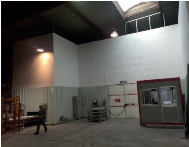
Enclosure of the transfer table aisle and the elevator and the lowerator ensure an energy-efficient system and protect the finger car.
