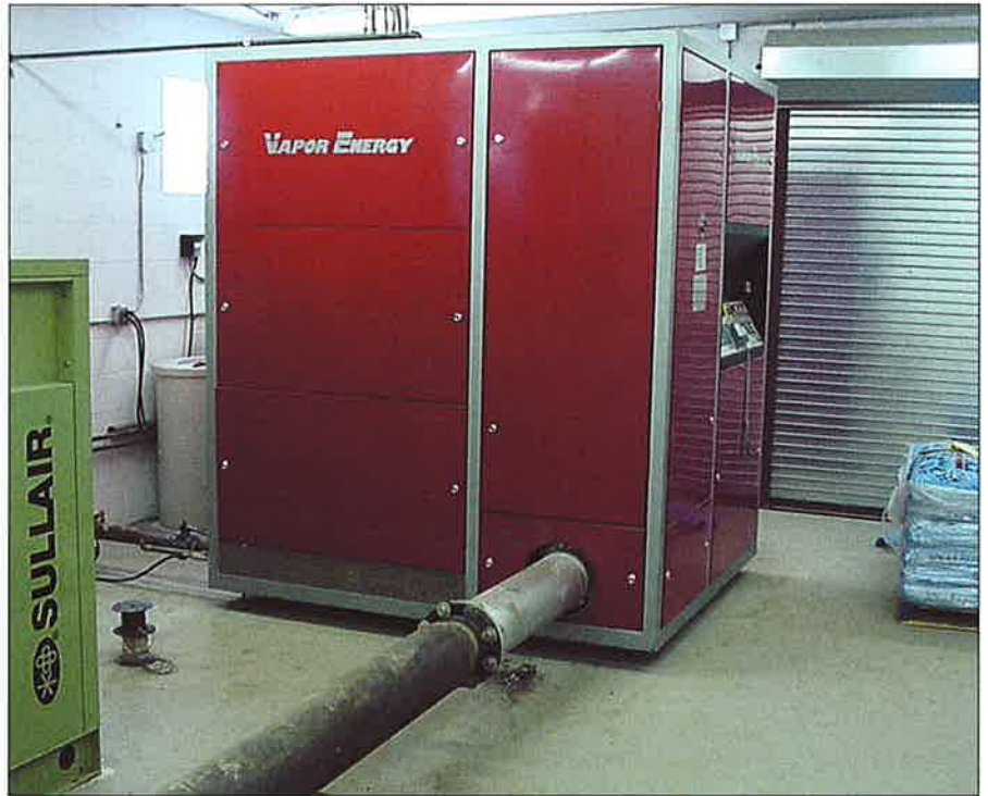
The cover of insulated sheet steel allows the plant to "whisper".
