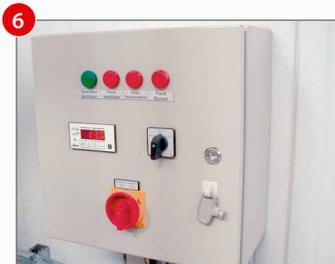
A simple two-point control system provides for automatic unsupervised temperature measurement and system control.
