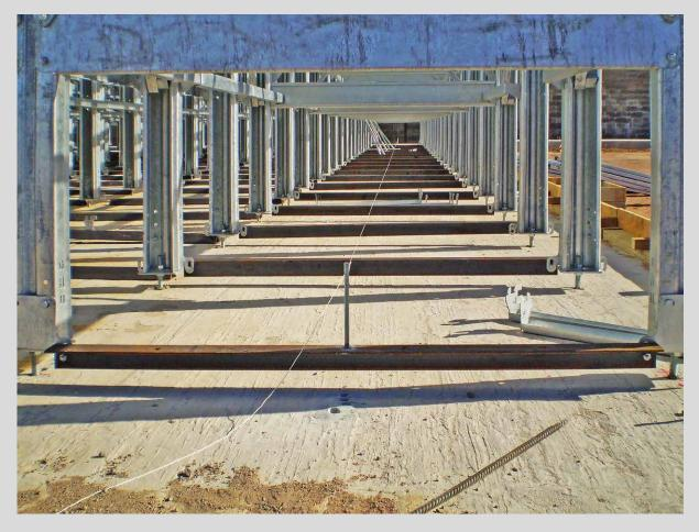
In traditional systems, the rack and rails have to be levelled seperately and each column must be levelled individually – a difficult and time consuming task. In addition, the rack and rails also have to be level to one another, a procedure that is imprecise and facilitates misalignment.
