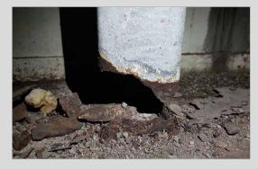
Due to condensation, columns close to the chamber wall are affected by corrosion while columns inside the chamber are not [picture on left]. Eventually, corrosion leads to complete failure of the column [picture on right]. The complete load-bearing structure needs to be replaced.
