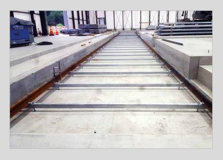
In existing rail systems, the rails are supported, connected and leveled with flimsy sleepers and concreted into place. During concrete works the sleepers and rails are easily displaced causing misaligned and unlevel rails.
