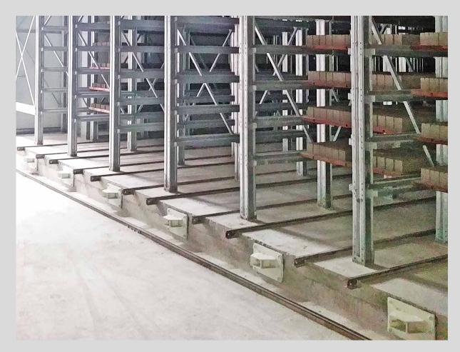
In existing rack systems, transport rails at the entrance of a rack passage tend to wear out as a result of constant stress. In addition, replacing the front portion requires excavating a portion of the concrete slab.
