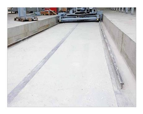
Only after concrete works are the rails installed either byweldingorwithclips. Rails are easily removed without concrete demolition and time loss.
