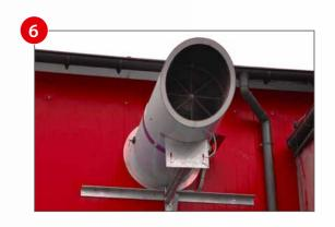
Our custom-designed exhaust system with electrically actuated damper (in order to prevent heat loss when not in operation) operates in order to reduce humidity.
