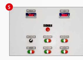
There are a wide variety of curing control alternatives available with our AutoCure® Automatic Curing Control System. It allows for temperature and humidity sensing, indication, controlling and, if required, recording.
