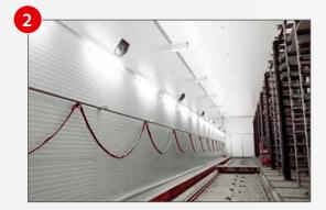
The NAUTILUS™ system prevents fog and condensation on chamber surfaces even at 35 °C (100 °F) and 90 % relative humidity. This prevents disruption of safety beams or control lasers and corrosion of the steelwork.
