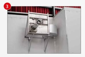
Our NAUTILUS™ radial ventilator is customer designed and manufactured for the concrete industry. Our stainless steel and aluminum construction and self-lubricating stainless steel bearing housing provide a durable solution in a harsh atmosphere.
