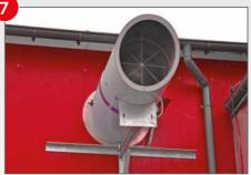
Our custom-designed exhaust system with electrically actuated damper (in order to prevent heat loss when not in operation) operates in order to reduce humidity.
