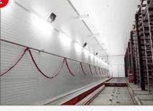
The QUADRIX® system prevents fog and condensation on chamber surfaces even at 35 °C (100 °F) and 90 % relative humidity. This prevents disruption of safety beams or control lasers and corrosion of the steelwork.
