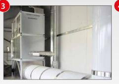
Our QUADRIX® unit is manufactured of stainless steel, aluminum and galvanized materials. Dual high performance radial ventilators provide high volume air circulation, while the 94% efficient heat exchanger is designed for efficiency and durability.
