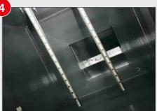
Our AutoFog® Moisture Addition System humidifies the air with finely sized steam fog in order to increase the relative humidity without drips, drops or the high maintenance associated with misting nozzles. The water is filtered softened and disinfected.
