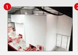
The rack is enclosed with insulated sandwich panels in order to reduce heat loss. Drawings and bills of materials supplied by KRAFT allow our clients a foolproof do-it-yourself solution for chamber insulation.
