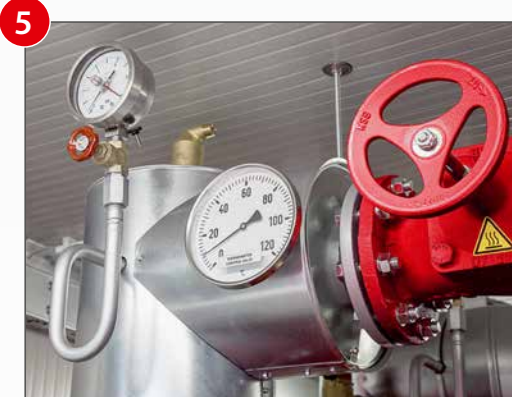
The system achieves a maximum concrete temperature of 50 °C to 70°C with water temperatures of 80 °C to 110 °C.
