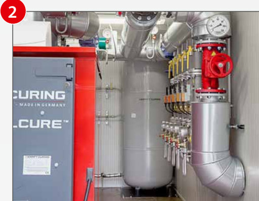
High-performance circulation pump available in bronze and stainless steel circulate the hot water from the water heater to the concrete form/mould/ table/bed and back.
