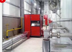
When compared to a boiler, the direct-fired vapor generator reduces operating costs by 40% to 60%. The vapor generator requires minimal space and operates at low pressure with propane or natural gas.
