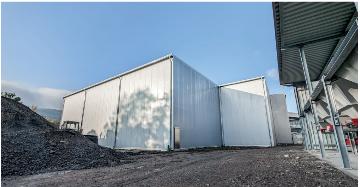
Modern curing chamber at Kraft Curing Systems GmbH in Germany
